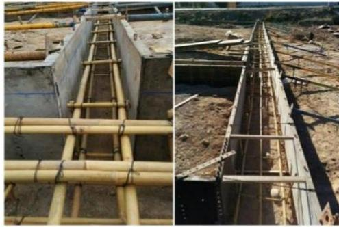
**Figure 1:** Bamboo reinforced concrete construction
