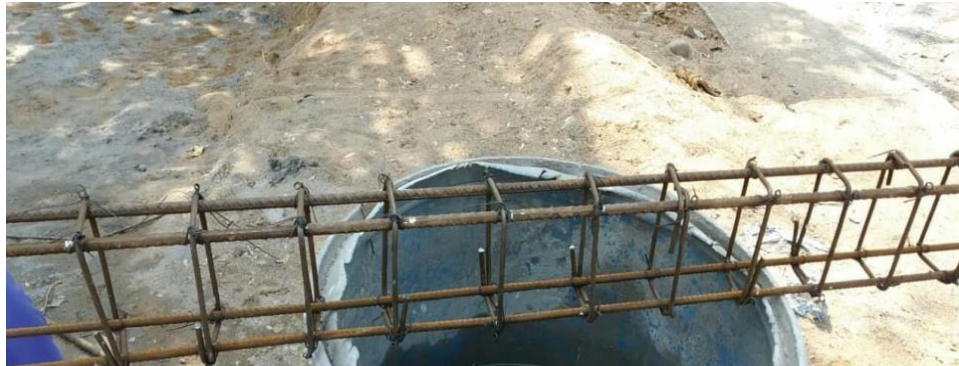
Figure 1: Conventional stirrups
