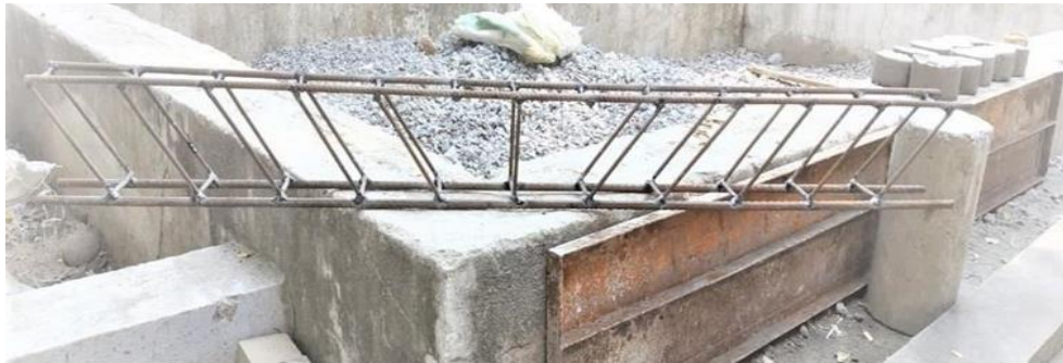
Figure 3: Rectangular welded swimmer bars
