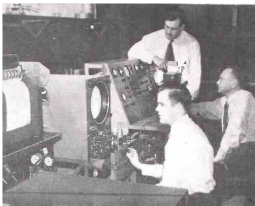
Figure 28. Dr. J Hillier in the foreground, Dr. VK Zworykin seated as well as R.L. Snyder with the early SEM, as published in the magazine Radio-Craft [132].
