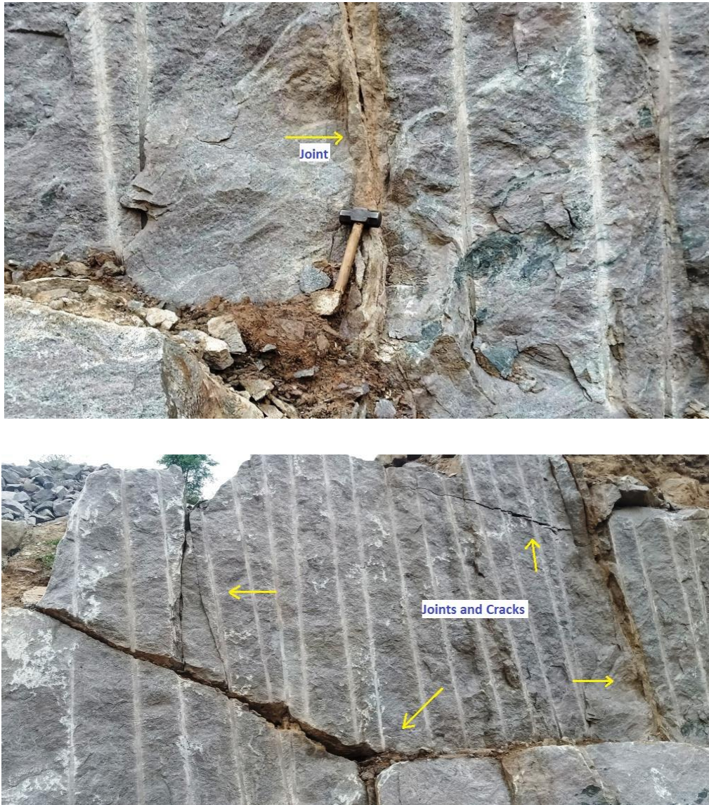
Figure 10. Joints and cracks, developed as primary origin or during quarry operations like blasting or at the time of dressing the block
