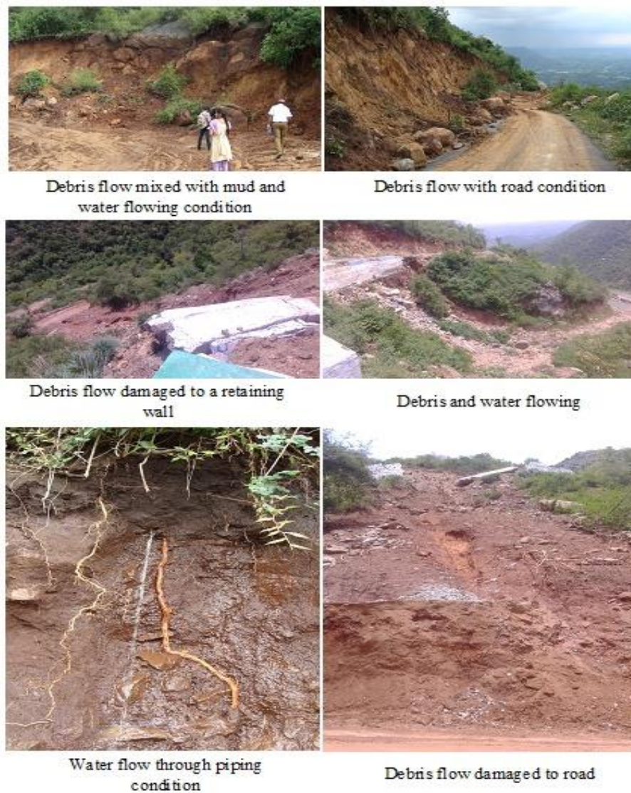
Figure 3. Field photographs show landslide inventory conducted at Debris flow site, Vathalmalai
