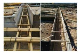
Figure 1: Bamboo reinforced concrete construction
