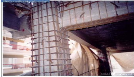
Fig: Concrete Jackting
