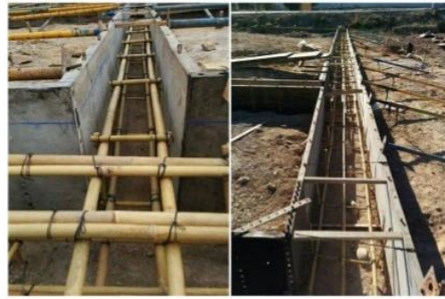
Figure 1: Bamboo reinforced concrete construction
