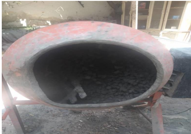
Figure 2.6.1 mixing of concrete
