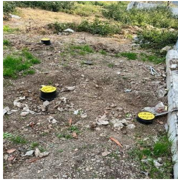
Fig.4: Double earthing
